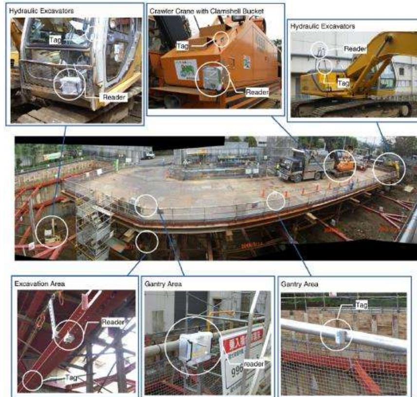
Fig. 4 Snapshots of construction site with RFID devices [45]
